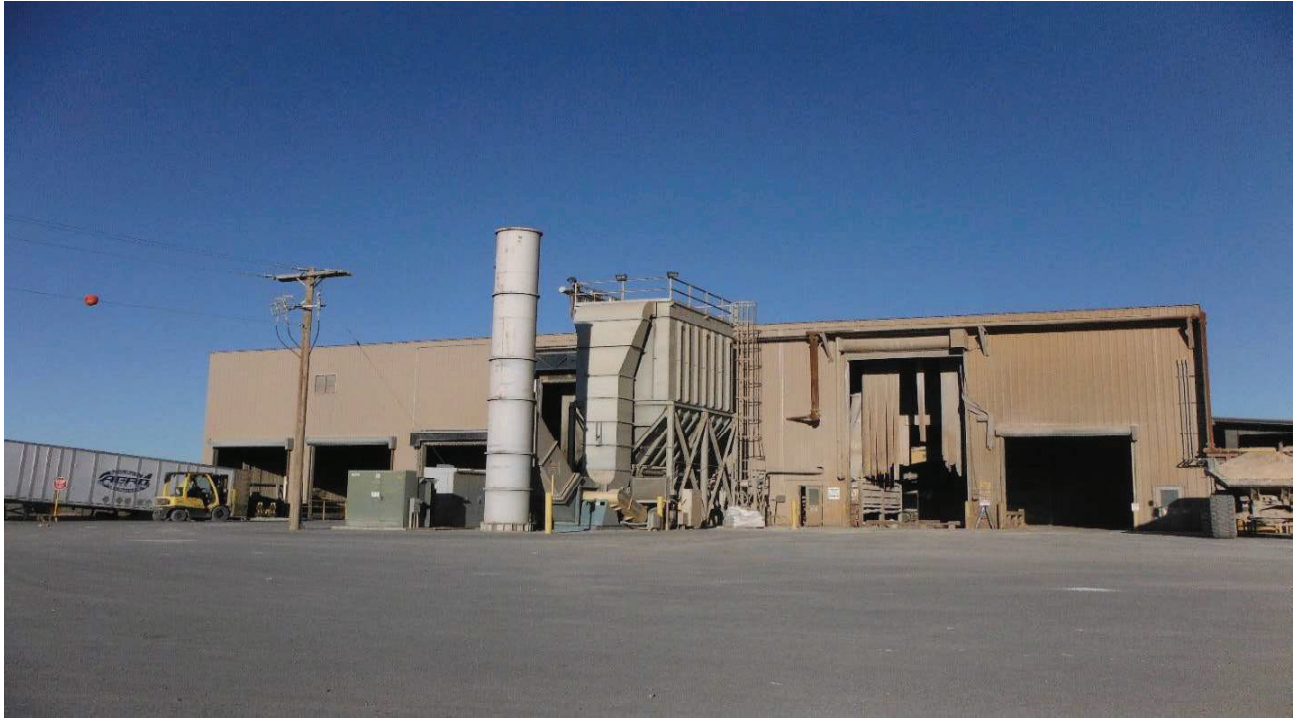
Photo 15- Tanks 18 and 19, aka Treatment Pans 4 and 5, with dust control baghouse in the middle. An unloading dock to Container Management Building 1 is on the left.
